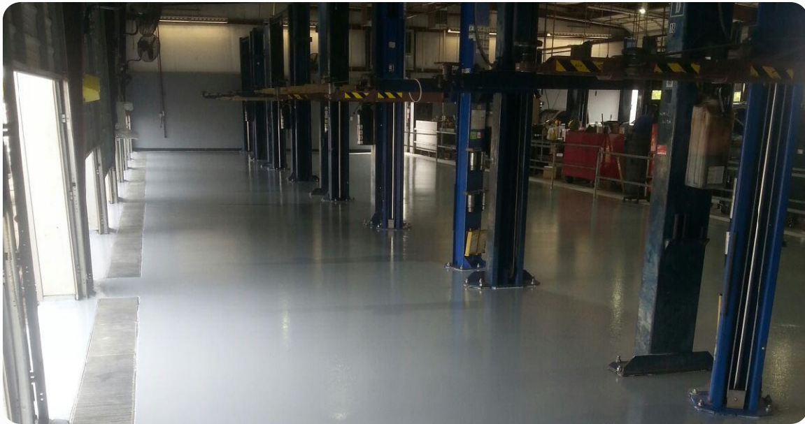
Photograph and installation by Sundek of San Antonio
