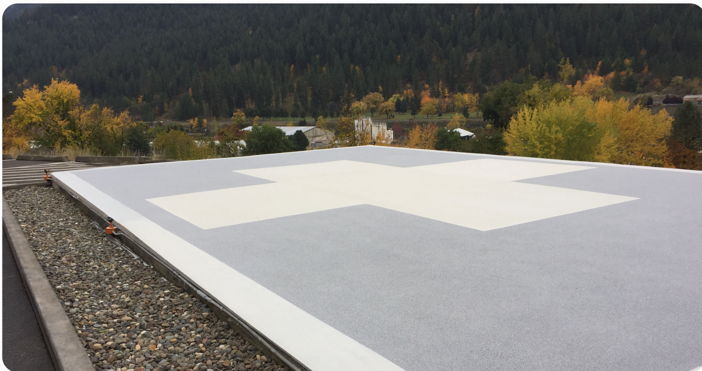
Photograph and installation by Knox Concrete
